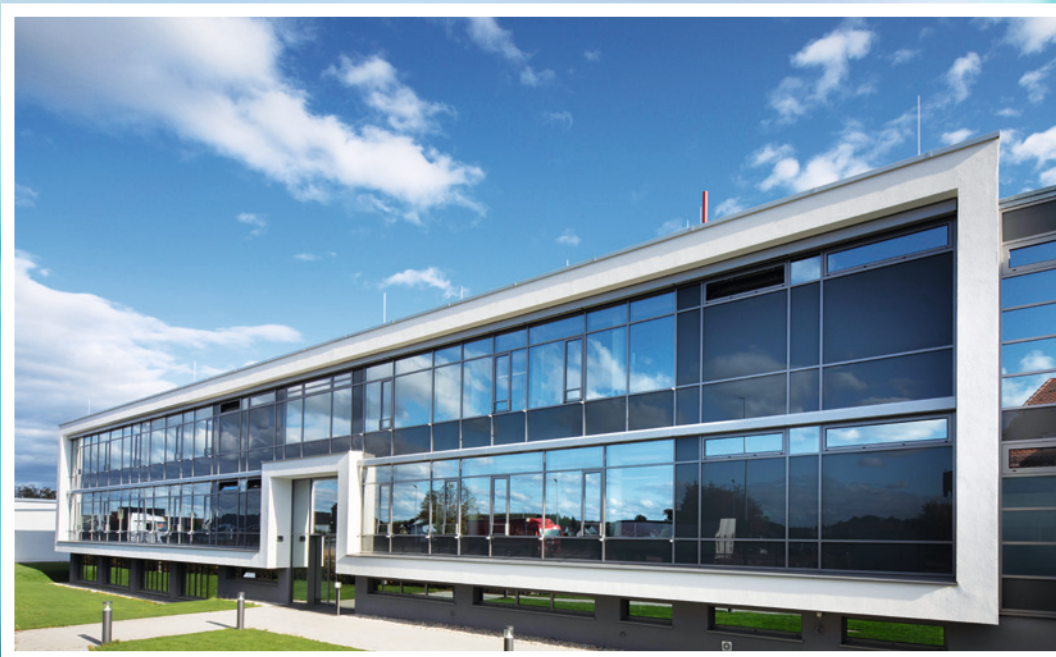
Company headquarters of Nabaltec AG, Schwandorf
